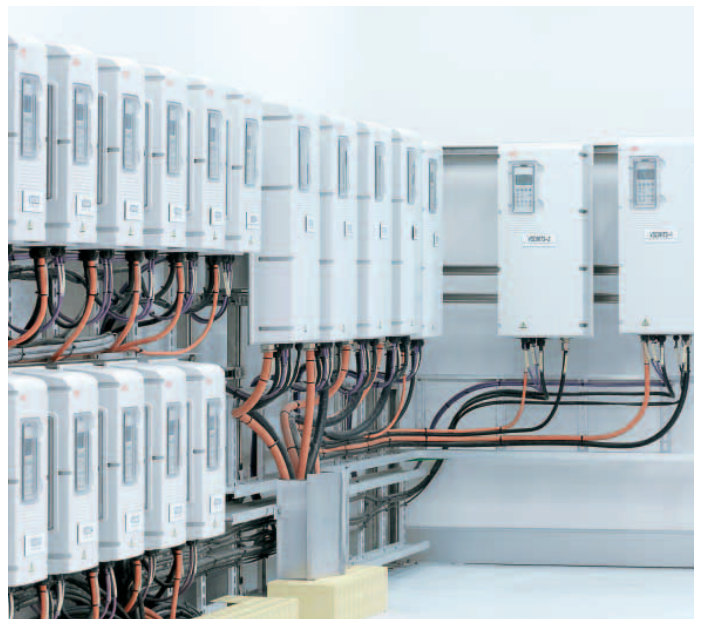
Among the built-in features of ABB drives are safe torque-off, EMC filters, brake choppers and drive protection.
